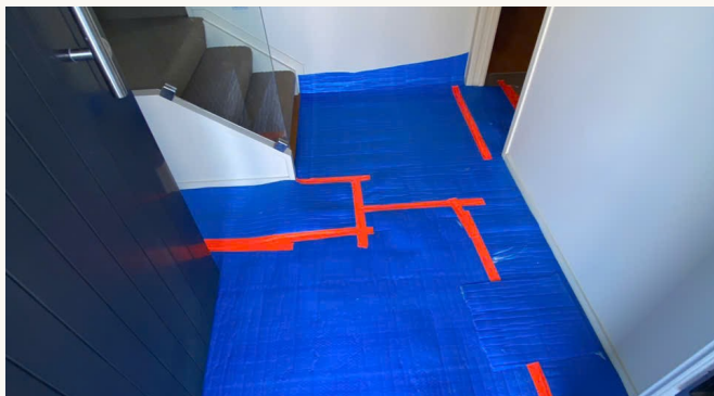
Protected route within a repair project | Onehunga
