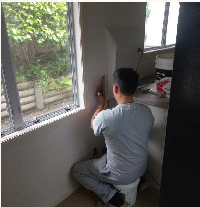
Wallpaper installation | Saint Johns
