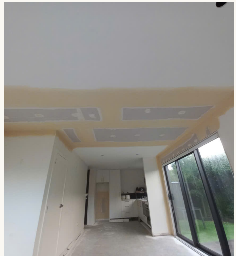
Te Atatu Peninsula | Broad ceiling preparation
