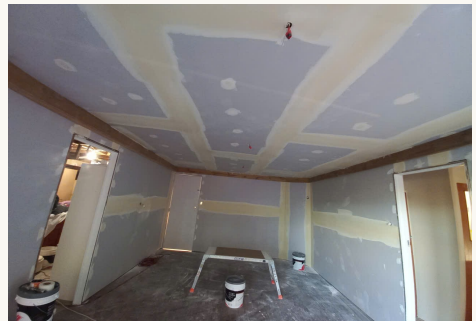
Plastering across ceiling and walls
