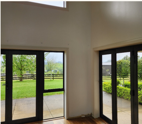
Dairy Flat | High interior surfaces
