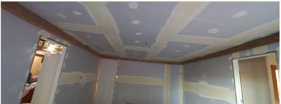
Maungaturoto | A broader reinstatement in progress
