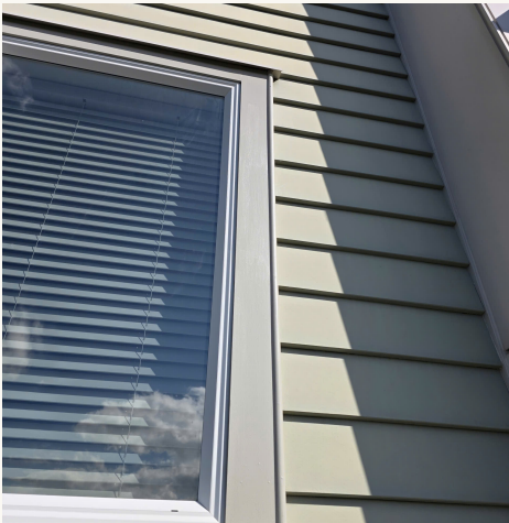
Stonefields | Window and weatherboard interface
