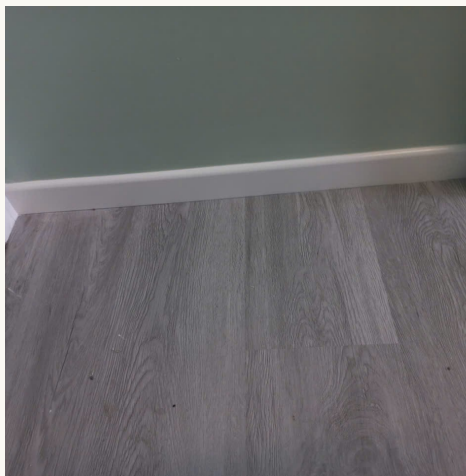
Te Atatu South | Painted skirting line
