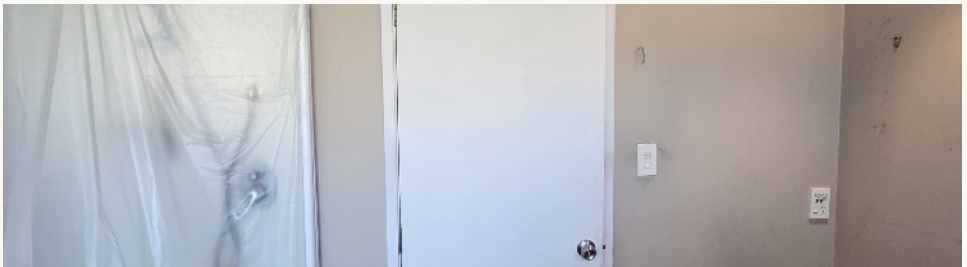
Wattle Downs | Wall repair and protection stages
