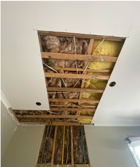
Ceiling opening and framing
