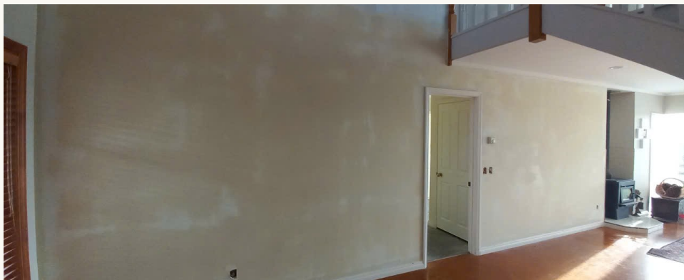
Pukekohe | Preparation before decoration
