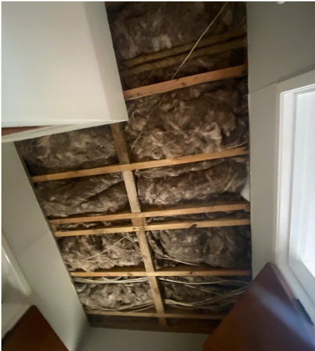
Maungaturoto | Exposed framing and insulation
