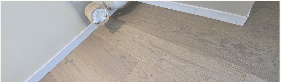
Wattle Downs | Wall and skirting detail
